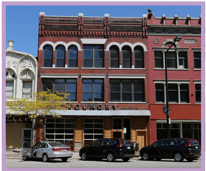
Figure 5.21 Historic, storefronts in downtown Elyria (Source: Cleveland.com)
