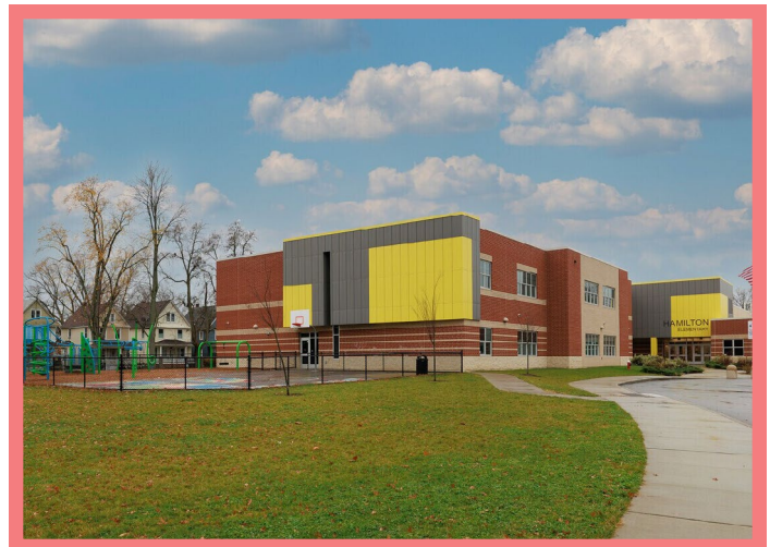
Figure 5.9 Hamilton Elementary School building, opened in 2022
