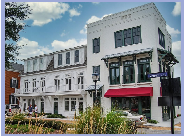
Figure 5.25 Townhomes and mixed-use apartments are types of housing units that can increase housing diversity in Elyria
