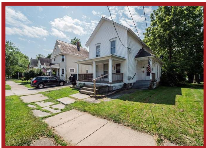
Figure 5.52 Sidewalks in disrepair along Middle Avenue (Source: Redfin)
